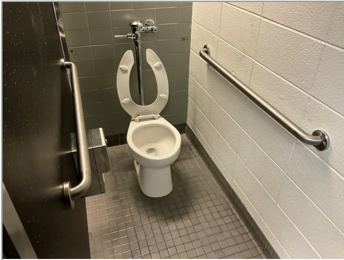
TOILET STALL OVERVIEW
