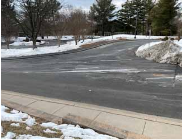
25 - SECONDARY PARKING AREA
