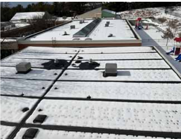
5 - PRIMARY ROOF OVERVIEW
