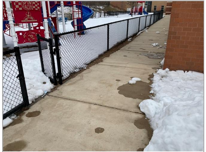
ACCESSIBLE ROUTE TO PLAYGROUND
