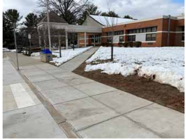
26 - SIDEWALKS AND LANDSCAPING
